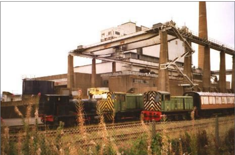
Below—Methil power station
