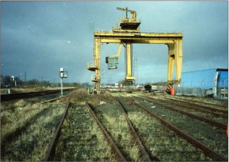
Above Portobello— old Freightliner depot -Morris crane still there.
