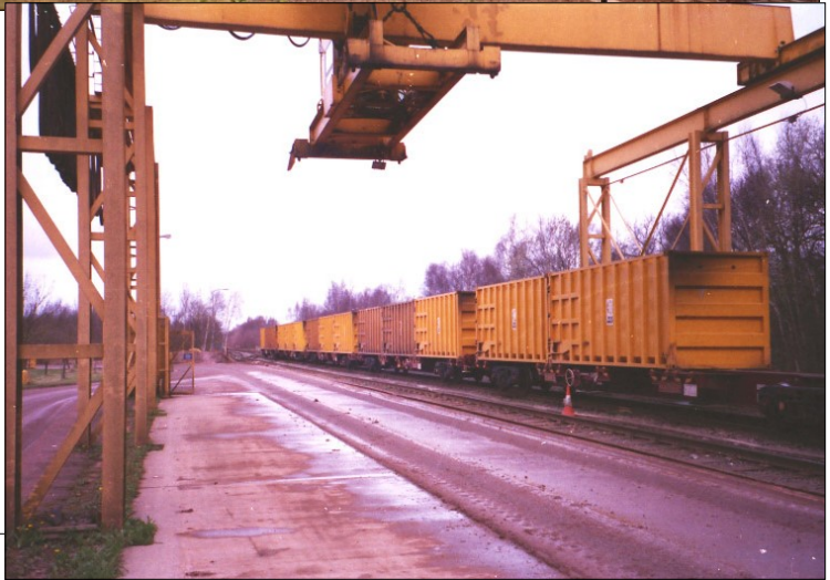
Left The closed diesel depot at Shirebrook West
