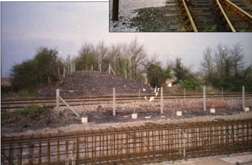
Below The “bridge” at Wentloog
