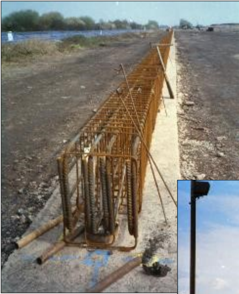
Above A new crane beam at Wentloog new terminal
