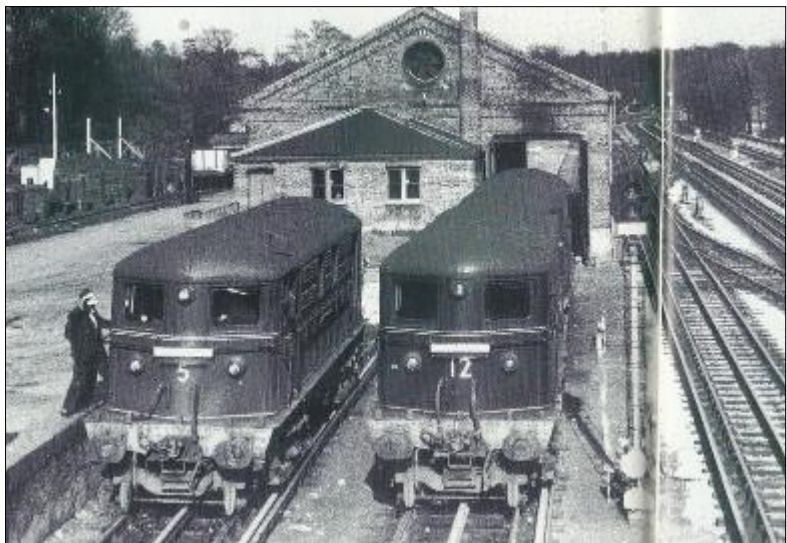
PHOTO A above. Fairburn 2-6-4T 42070 moves forward to couple onto an Aylesbury-bound train while "Growler" No 18 Michael Faraday, which has just brought the train from Baker Street, returns to the electric loco stabling sidings via the up line. PHOTO B below Metrovick Locos No. 5, John Hampden and No. 12 Sarah Siddons (now preserved), together with a third unidentified loco, stand in the electric loco stabling sidings circa 1960. Photos courtesy author.
