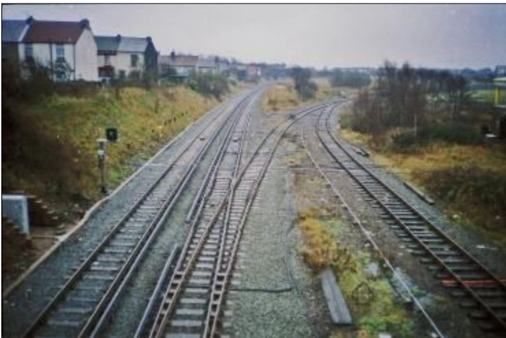
Aintree Station Junction with the Noryth Mersey branch.
