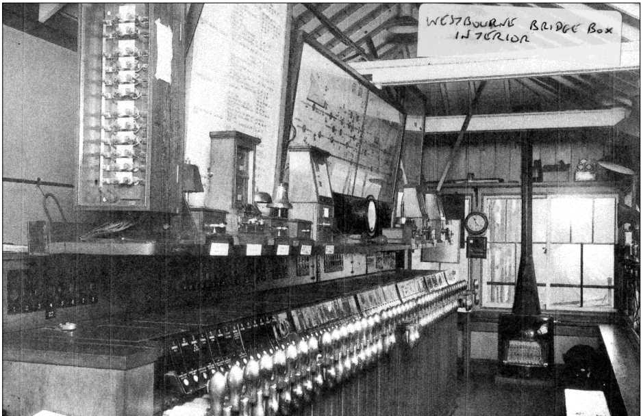
Westbourne Park box interior.
