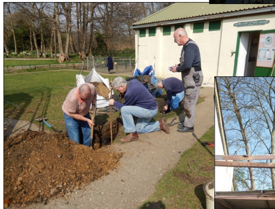
Above Club house drainage replacement.
