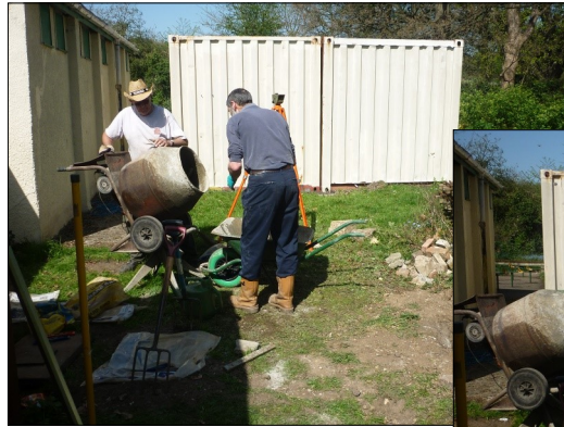
Above Hard standing for the container being laid.
