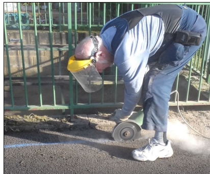
Right Nigel Penford doing the horribly messy and back breaking job of disc cutting the trench across the tarmac.
