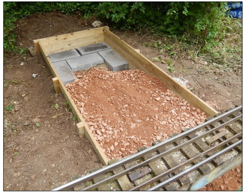
Above. Raised track progress Left top. Cutting the Baldwin axle.
