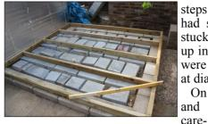
steps are still very solid even when wet. I had some heavy duty blocks so these got stuck down and some lighter ones got used up in the middle. Carefully measured beams were placed and screwed next. Lily is good at diagonals.
