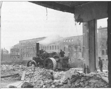
To accompany the article from page 3 by John Spokes this is a rare Fowler class AA3 ploughing engine being used in 1953 to pull out pipes and beams from the rubble of the Mobius department store in Dresden. This photograph was taken by Mr Mobius himself no doubt wanting to record every step of the demolition of his bomb damaged store. Photo University of Dresden Library and courtesy of the Steam Plough Club.
