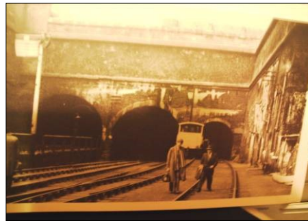
A VIEW OF THE THREE TUNNELS- THE ONE WITH THE HORSE TROUGH IS ON THE RIGHT Also note one of the special six wheeled brake vans waiting its train
