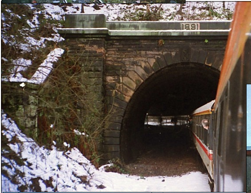
Left below, Totley Hill tunnel
