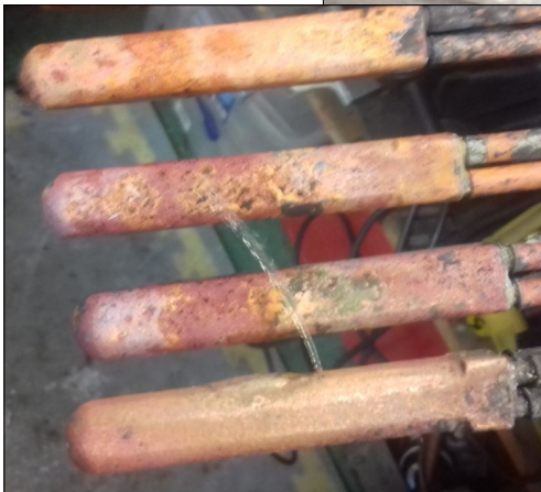
The leaking superheater from Nigel's engine.
